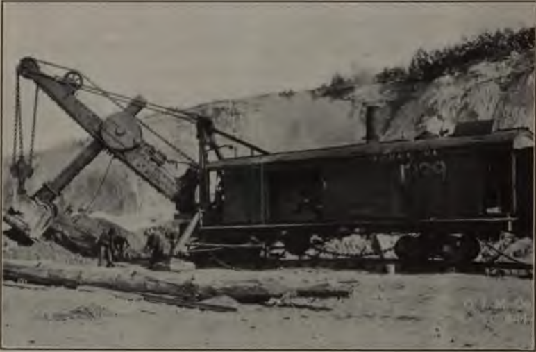
No. 11—Canisteo Pit, Steam Shovel, Coleraine, Minn.
